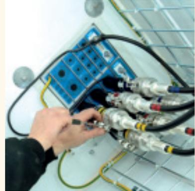
Picture 4: Installation of communication cables
